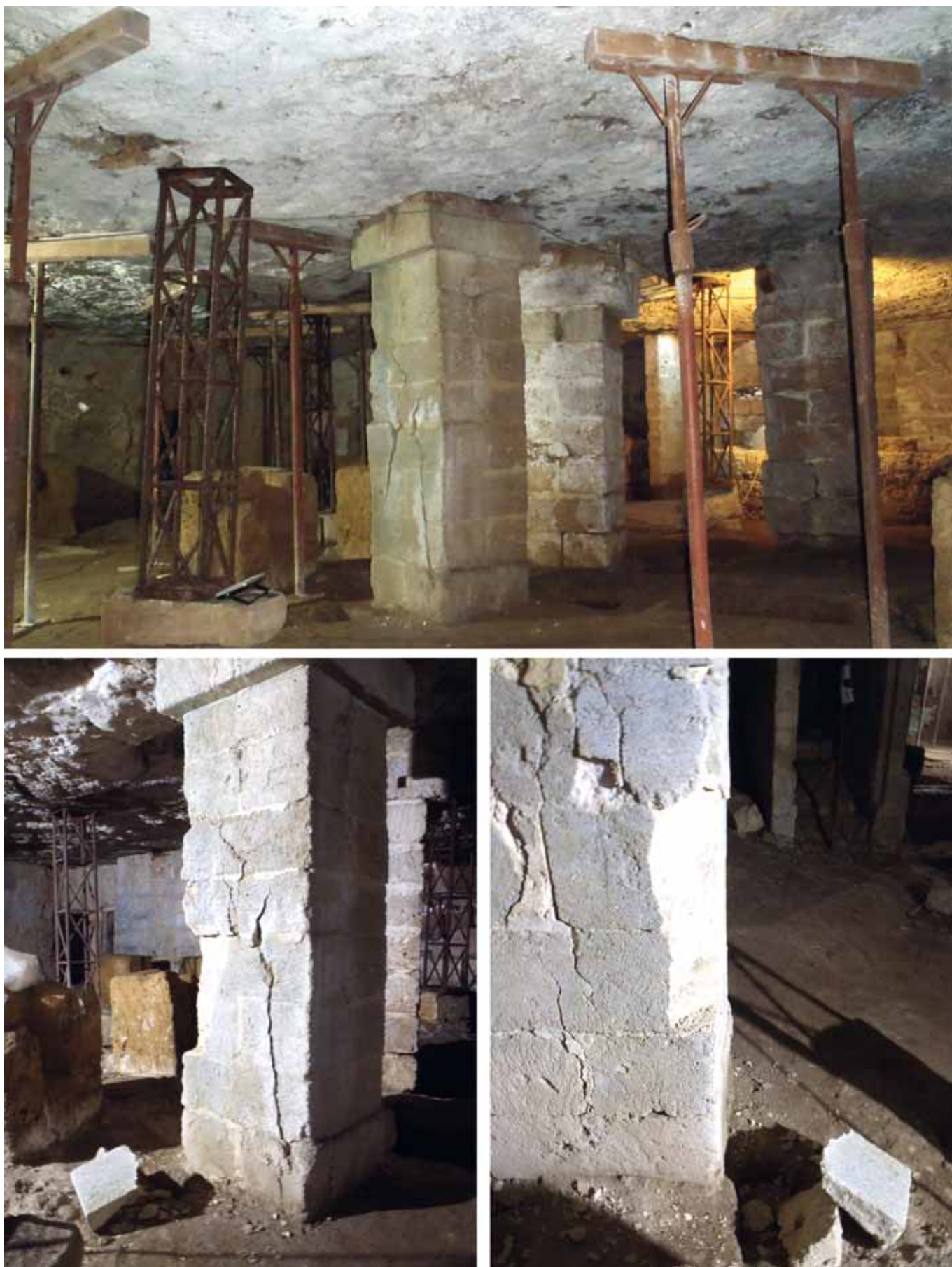
Fig. 8 – General view of an underground oil mill affected by serious fracturing, and details of a fractured pillar, from which detachment of small parts of rock has already occurred, due to excessive overload (photos: M. Parise).
