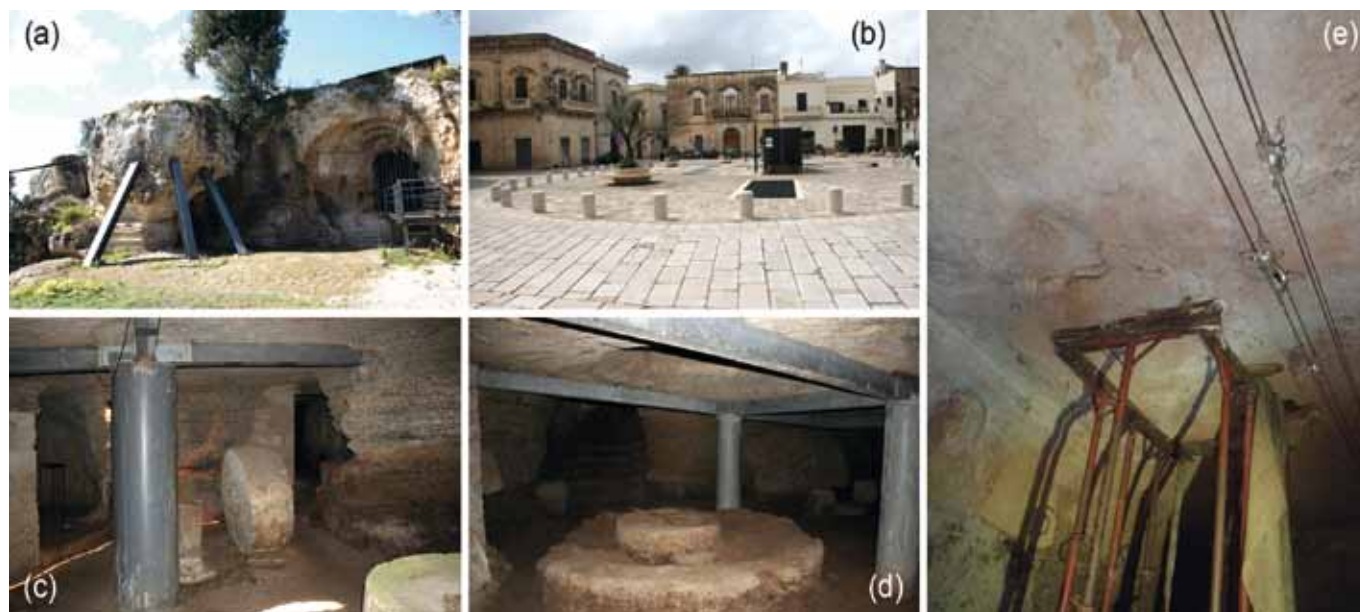
Fig. 9 – Stabilization works in artificial cavities of cultural heritage in Apulia: a) sustaining steel rods at Fasano; b) view of the main square in Presicce, showing the entrance to the system of underground oil mills; c, d) details of piles and beams for stabilizing the site, that is now open to public; e) temporary scaffolding to sustain the vault, showing open cracks, at Cantina Spagnola, the most famous artificial cavity of cultural interest at Laterza (photos: M. Parise).
