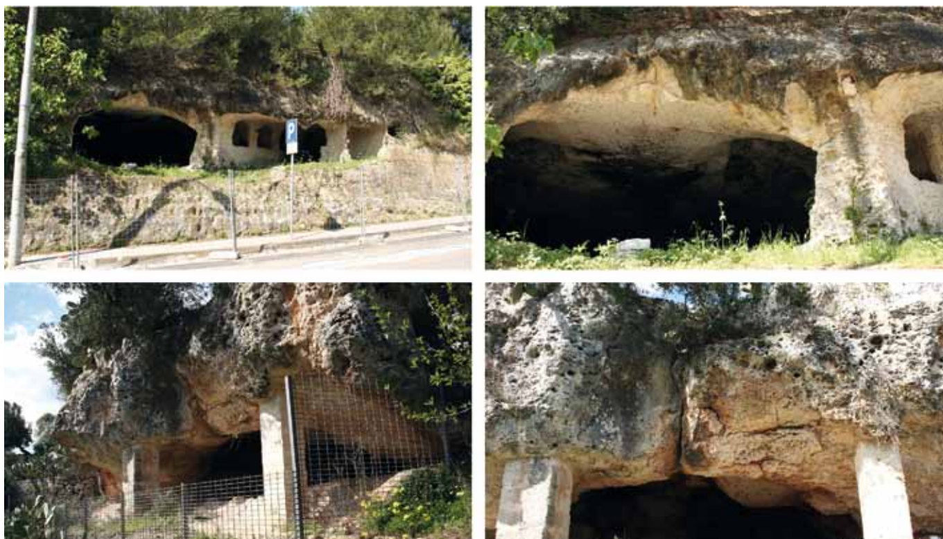
Fig. 5 – Open cracks crossing the entrance of artificial cavities, threatening the overall stability of the sites: above, artificial cavities at Otranto; below, a cavity in the Fasano area (photos: M. Parise).
