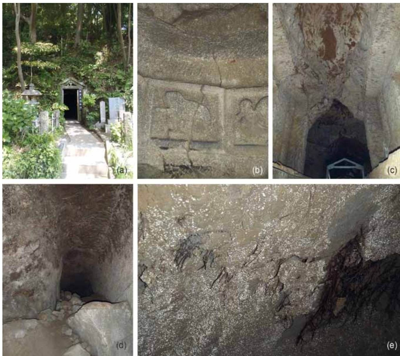
Fig. 7 – Taya Cave, Japan: a) entrance of the cave; b) cracks crossing some reliefs on the walls of one of the meditation chambers; c) evidence of slab detachments from the vault; d) fall deposits of variable size partly closing a sector of the cave; e) roots entering the wall cave, causing exfoliation processes in the outer portions of the rock mass (photos: M. Parise).
