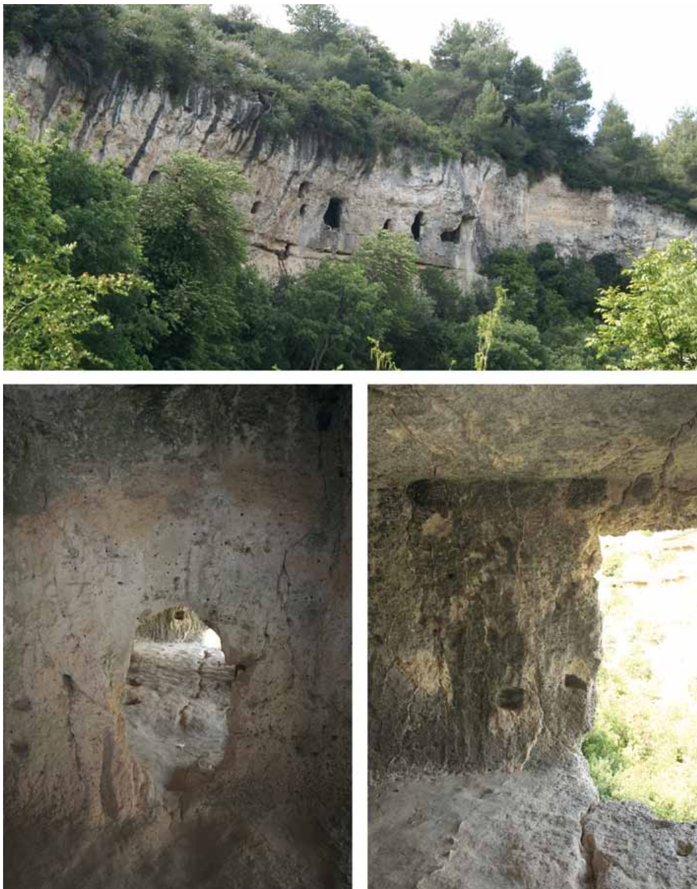
Fig. 2 – Farmacia del Mago Greguro ( Wizard Greguro Chemist's ), a well-known artificial cavity excavated along the flank of a karst valley at Massafra (Apulia, Italy): above, general view of the site; below, release tension cracks extending from pavement and walls to the vault in the outer part of the cave (photos: M. Parise).
