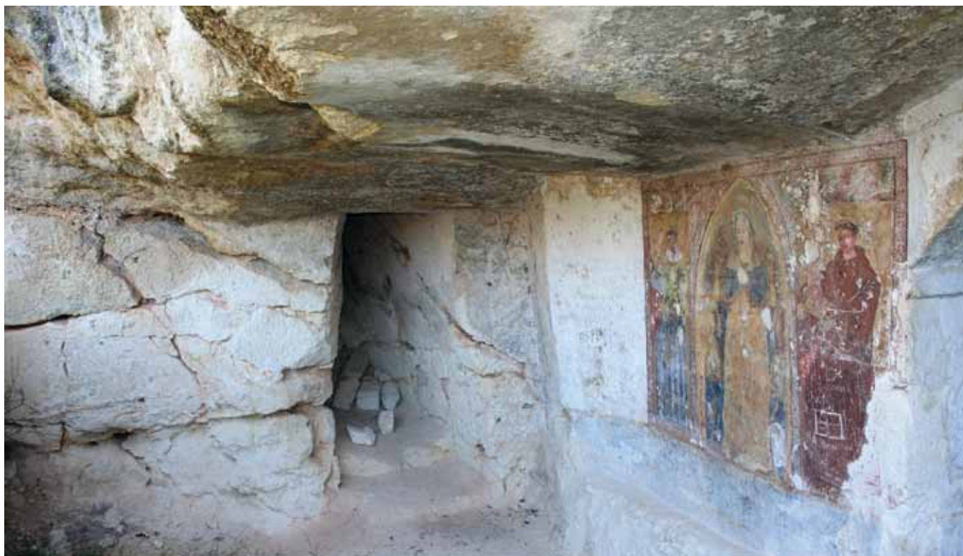
Fig. 4 – Severe cracks affecting a worship site (typology of artificial cavity C1 in the classification by Parise et al., 2013) (photo: M. Parise).
