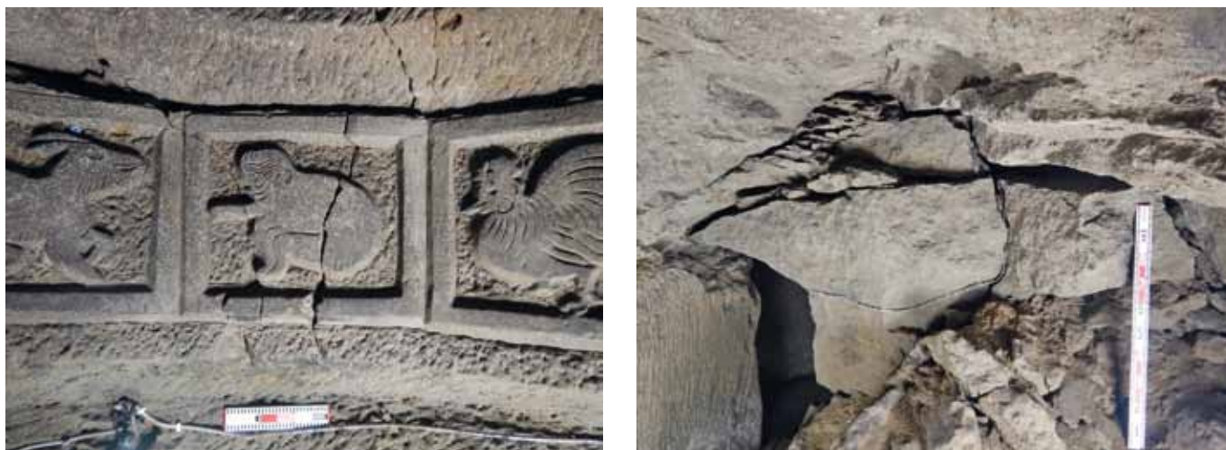
Fig. 8 – Some images acquired in the Taya Cave. From the images, it is possible to figure out that there is a very critical situation with structural failures in progress. Collapses can occur at any moment, putting visitors at risk (photo: ISASI/CNR©).
