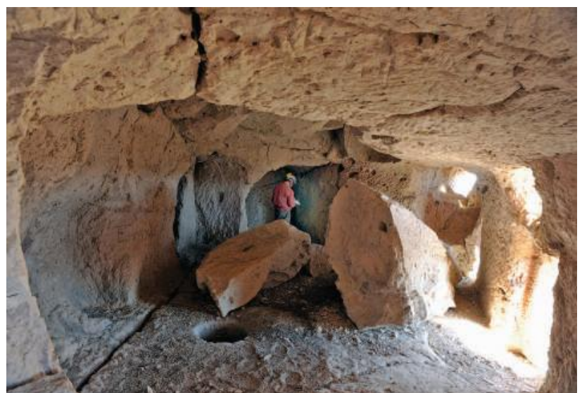
Fig. 11. Şahinefendi. Rock-cut dwelling and shelter of Orta Tepe (Ne71.1). Upper floor with evident cracks and falls, in imminent danger of further collapse (photo Bixio A.).
