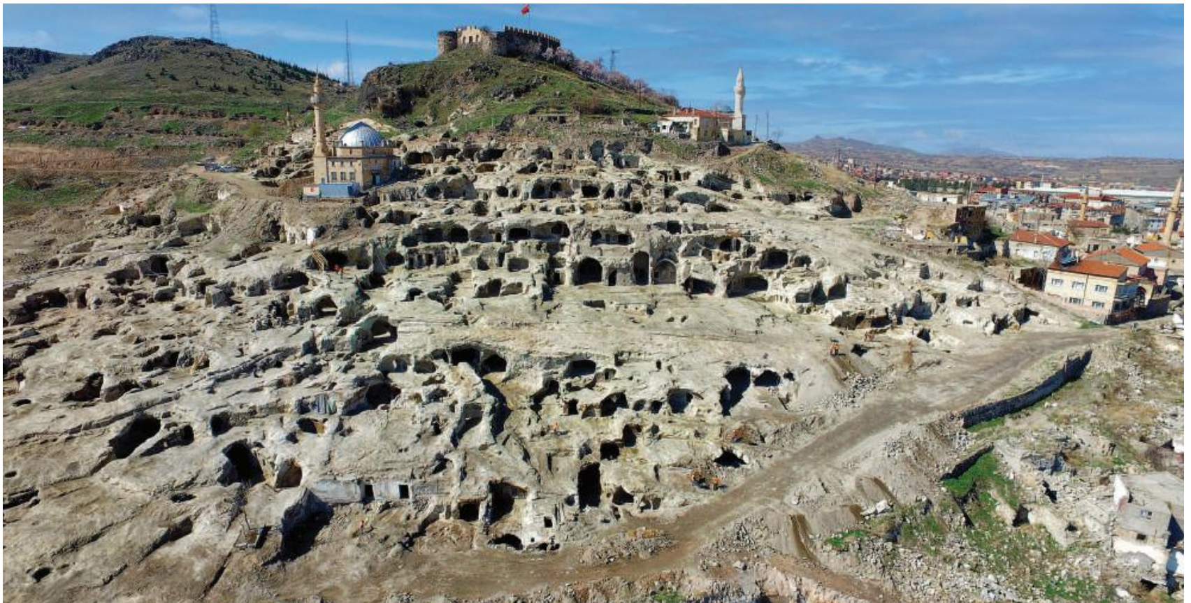
Fig. 3. Nevşehir. The “terraced” rock-cut village (Ne73.1), unearthed in 2015 (photo courtesy Gülyaz M.).
