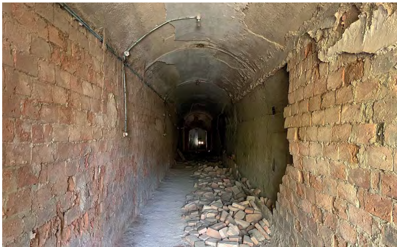
Fig. 5 – View of the tunnel from the entrance. In evidence, the masonry partition wall used for creating the air shaft, partially collapsed as shown in the right side of the photo (photo M. Cangemi).
