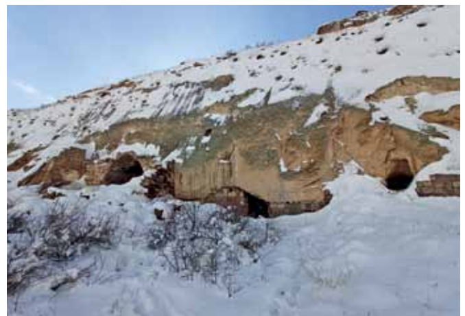
Fig. 4 – Entrances of Derevank Monastery rock-cut complex. Harsh winters (up to 25 degree below zero), and hot summers, are probably the earliest reason that pushed the inhabitants to take advantage of the thermal inertia that characterizes the spaces excavated into the cliff (photo A. Yamaç).
