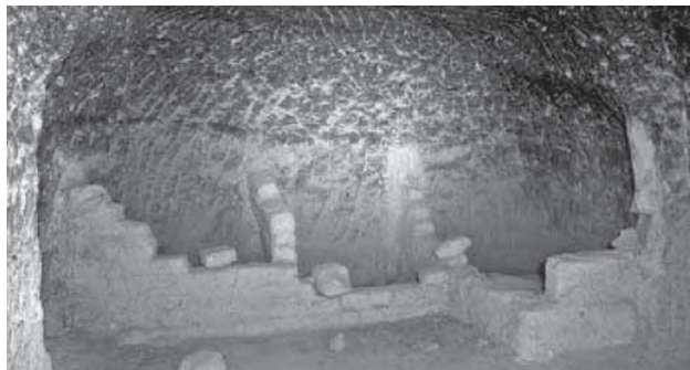
Fig. 9 – Masonry of adobe bricks inside the rooms allocated the compartments. Traces of tools on the walls are clearly visible (photo N. Moldavskaya).
