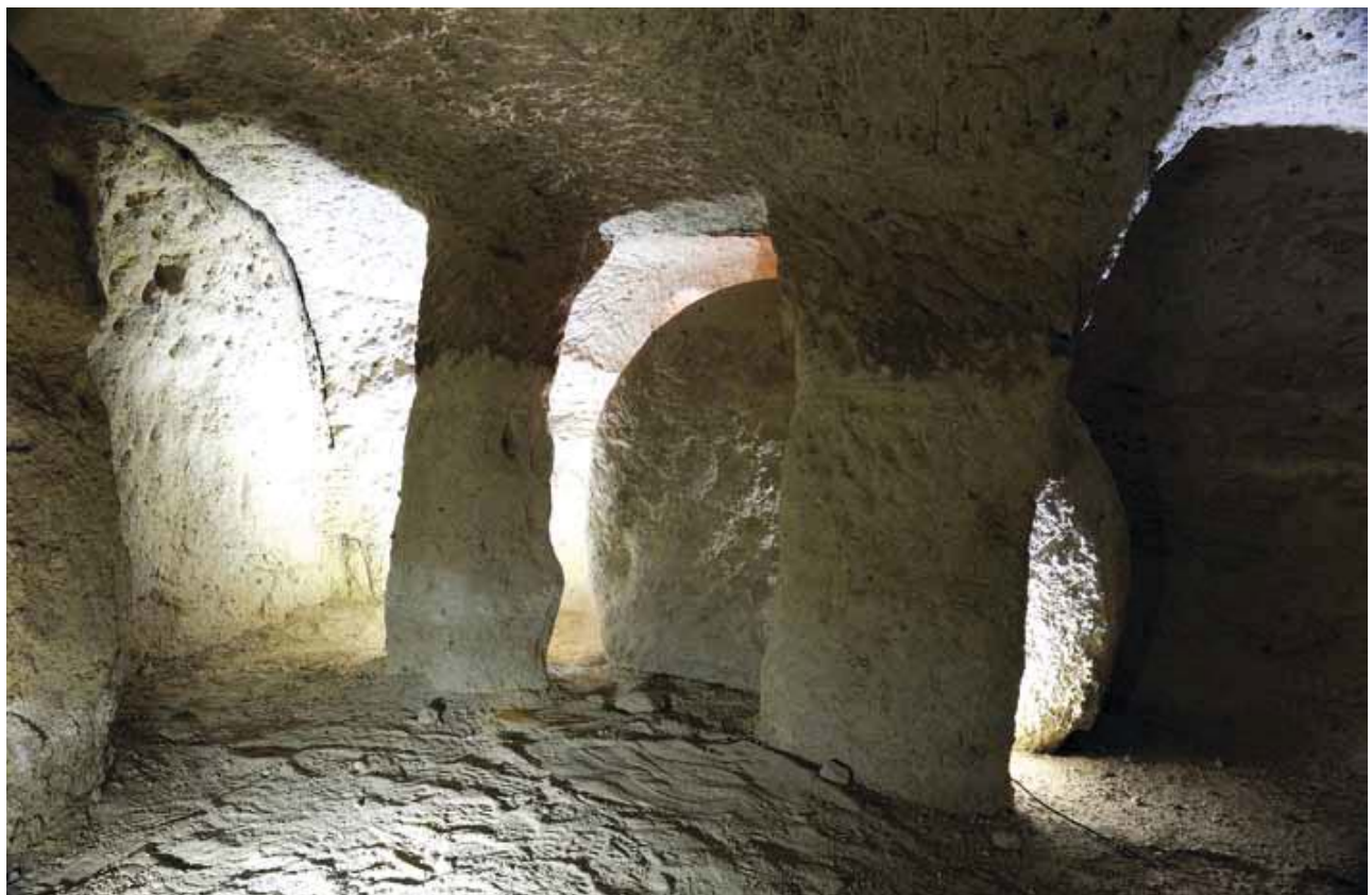
Fig. 20 – St. Eustachius shelter. Millstone-door and support pillars (photo A. Bixio).
