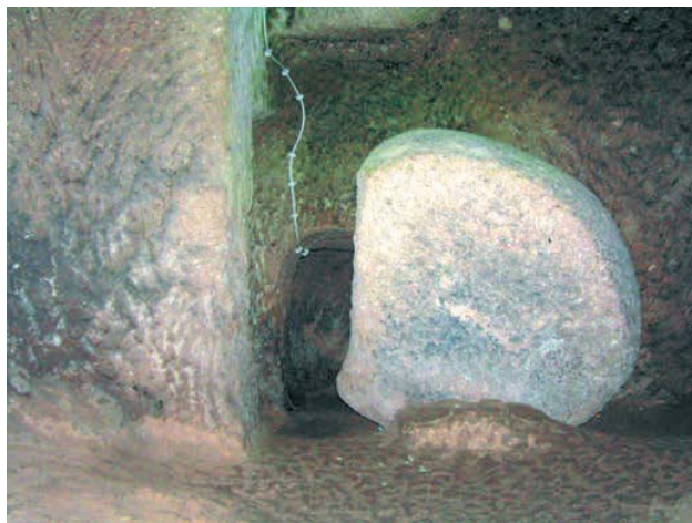
Fig. 9 - Closing device (millstone-door and support pillar), partially destroyed, in room 24 (photo A. Kovalev).
