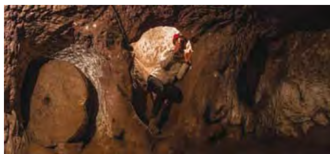
Fig. 6 - First mill stone door after the entrance of 4. Underground Structure (photo C. Cankirili).
