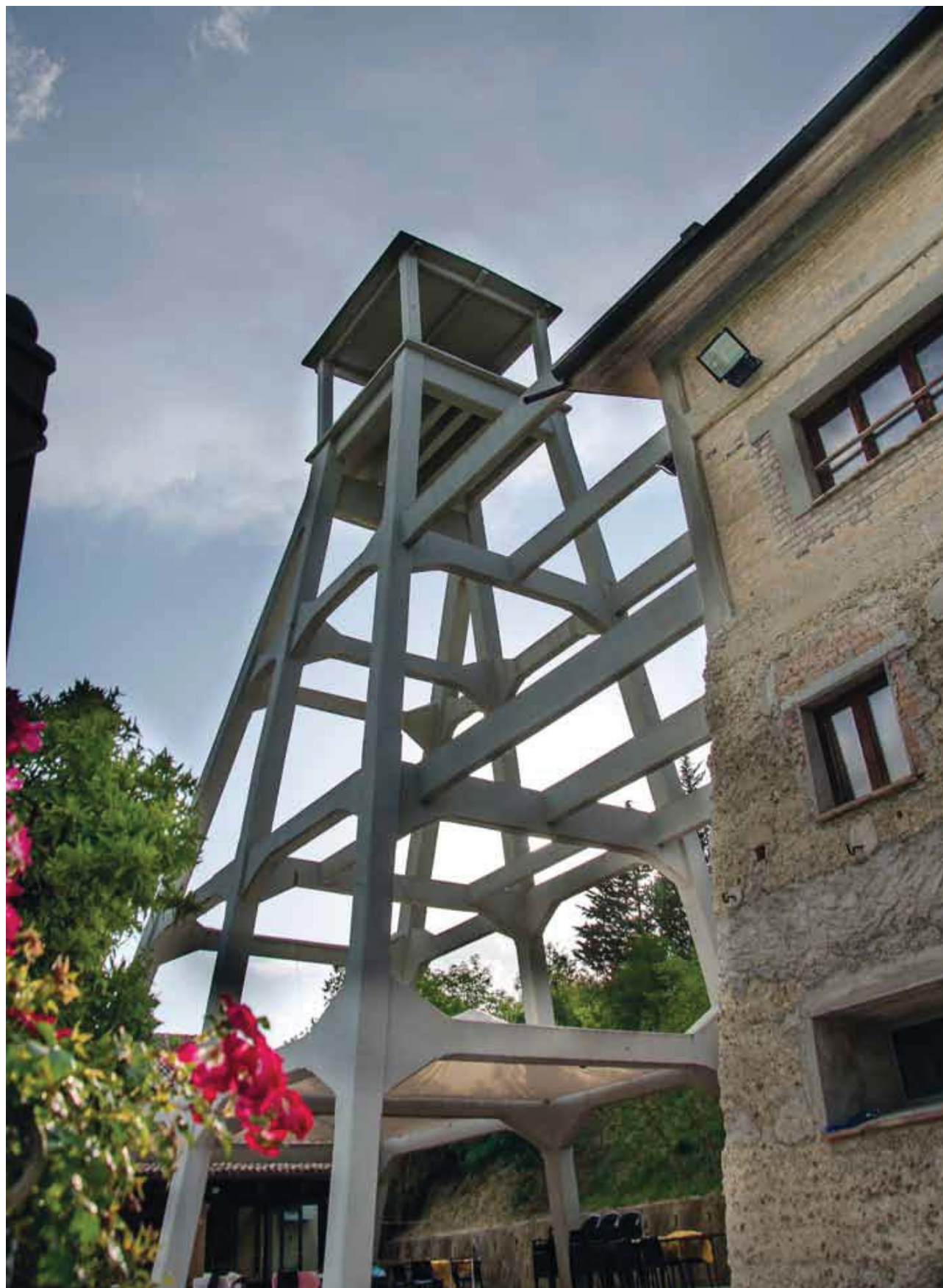
Fig. 9 - Castello in cemento armato di servizio a Pozzo Donegani (foto E. Diakatos A.). Fig. 9 - Castle in reinforced concrete service at mine pit Donegani (photo E. Diakatos A.).
