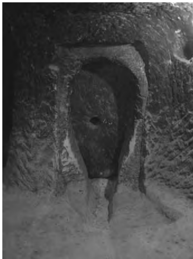
Fig. 14 - Closed mill stone door of the east tunnel of third floor (photo: A. Yamac).
