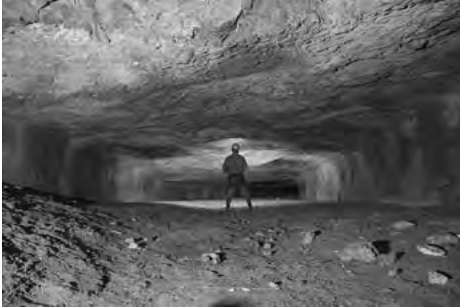
Fig. 5 - Deviation Tunnel. The ground is filled with sediment thicker than 2 meters (photo: E. Gilli).
