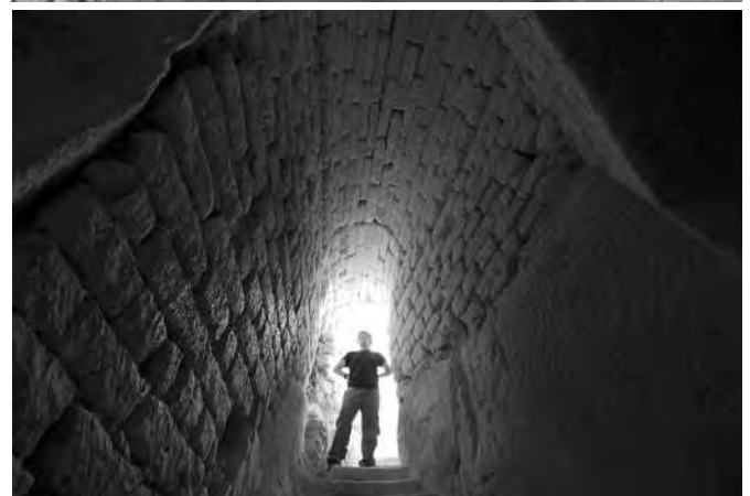
Fig. 32 - A) SC 53 - photo of constructed vaulted dromos leading to cistern no. 1 in fig. 29; B) Photo of the vault, made of chalky limestone blocks(photo B. Zissu).
