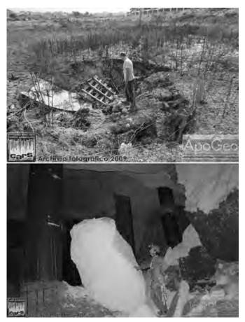
Fig. 3 - A sinkhole at Altamura, and an example of the failures in the underground system of quarries (photos by Centro Altamurano Ricerche Speleologiche).
