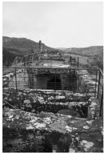
Fig. 6 - Fleckenstein: view of several rock-hewn (open to the sky) cellars situated just below the top platform.
