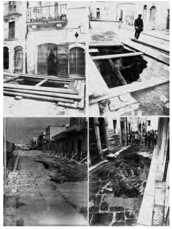
Fig. 5 - Sinkhole events in the urban area of Andria (photos dating back to the early '70; source: Basin Authority of Apulia): above, via Federico II di Svevia; below, via Pietro I Normanno and via C. Colombo.
