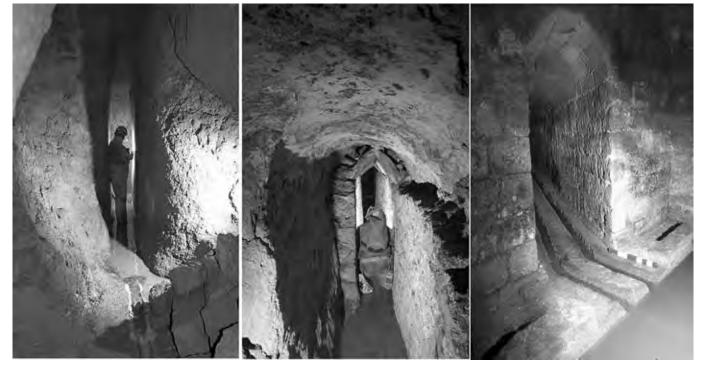
Fig. 5 - Examples of underground aqueducts: a) ancient aqueduct, re-worked in the XVII century by monks of the Camaldoli Hermitage at Mount Tuscolo (Latium); photo archive Egeria Centro Ricerche Sotterranee; b) branch of the late roman aqueduct at Roccarainola (Campania), realized in pyroclastic deposits; photo F. Maurano; c) channels within the aqueduct Fontana della Stella at Gravina in Puglia (Apulia); photo G. Bologna.
