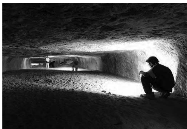
Fig. 22 - Ancient tunnel excavated to divert the Kızılırmak River (photo A. Bixio).
