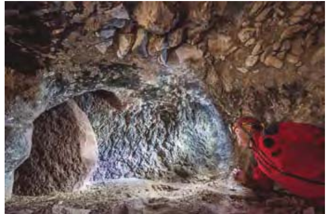
Fig. 14 - Mill stone door of Otedere Valley Underground City No 1 from the operation room (photo A.E. Keskin).
