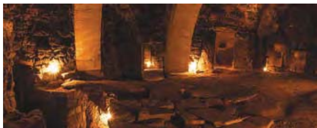
Fig. 13 - Main chamber of 4. Underground Structure with a barrel vault roof (photo C. Cankirili).
