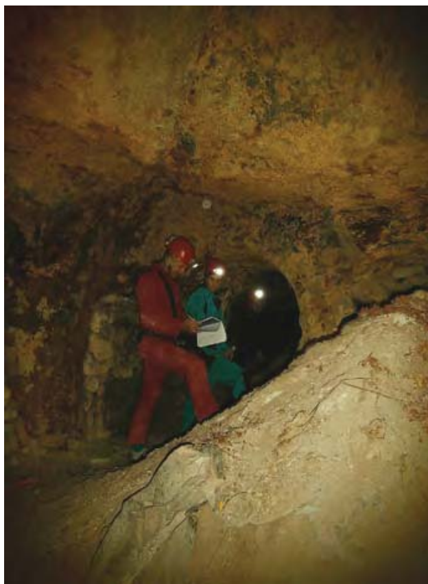
Fig. 16 - One of the abandoned rooms in the last part of 4. Underground Structure with debris from the roof (photo A. Yamac).
