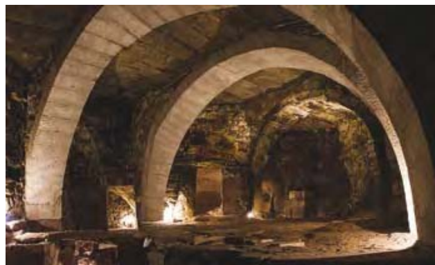
Fig. 8 - Third chamber of 1. Underground Structure with a barrel vault roof. The farthest vault is an original 15. century structure, two front ones are contemporary restorations (photo C. Cankirili).
