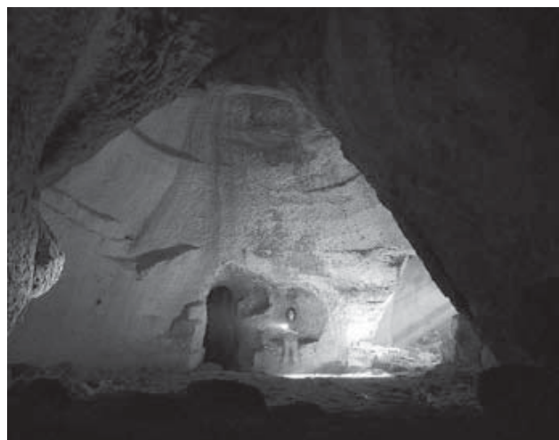
Fig. 6 - Parallel rows of oblique chisel marks on the walls of a bell-shaped cave at H. Burgin (photo B. Zissu).
