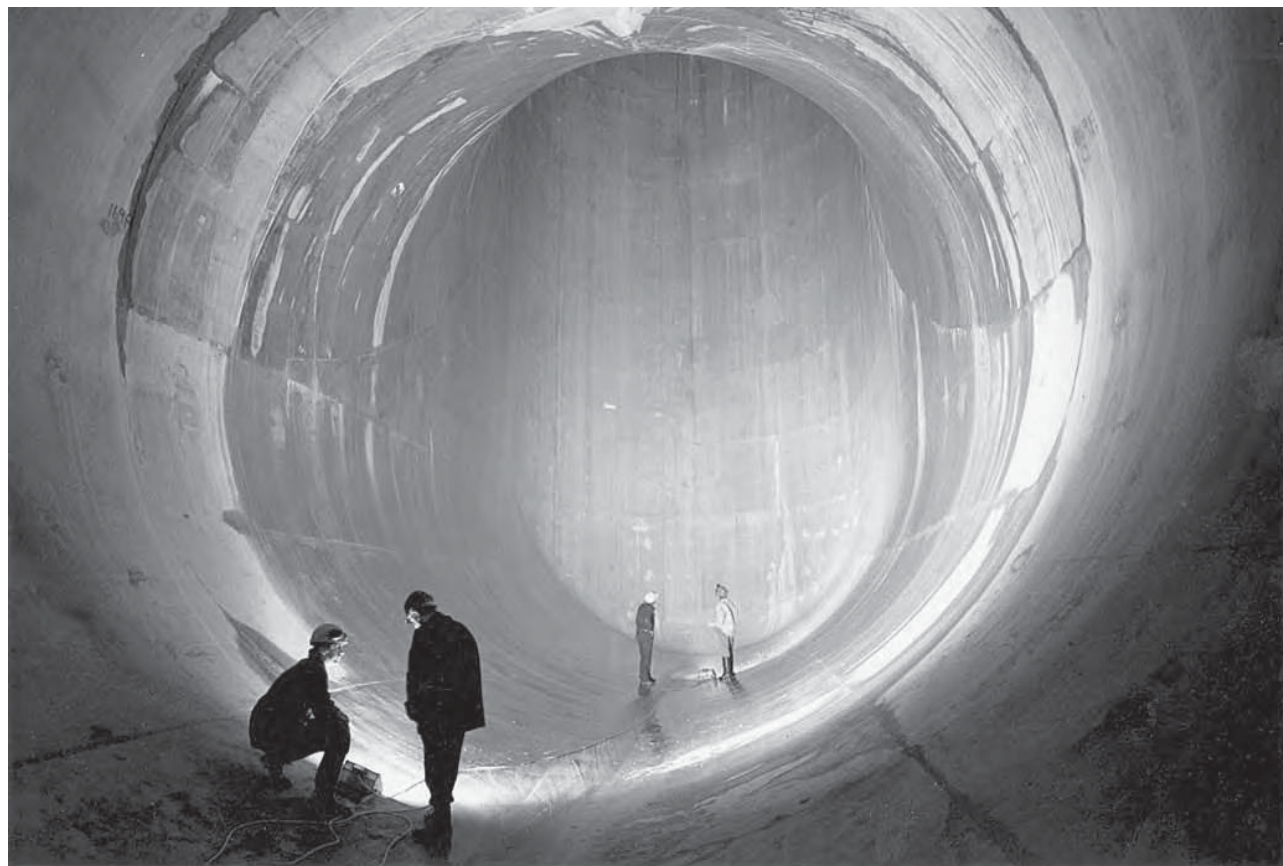
Fig. 15 - Surge tunnel at Dinorwig Hydro-Electric power station (photo First Hydro Company).
