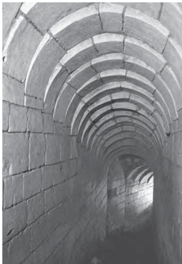
Fig. 12 - The access corridor of the village underground refuge of Filescomp, region of Arras; the vault is characteristic of the underground refuges of Northern France. Height: 2 m (photo J. & L. Triolet).
