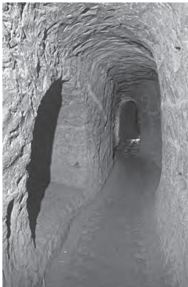
Fig. 16 - Central gallery that gives access to rooms located on each side, intermediate level of the village underground refuge of Vinh Moc, Vietnam. Height: 1,80 m (photo J. & L. Triolet).
