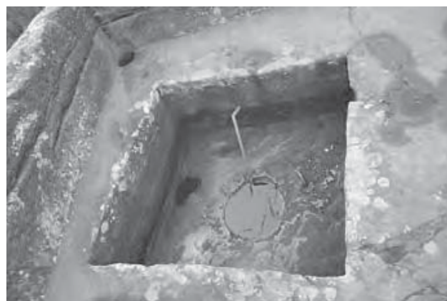
Fig. 13 - Drachenfels: filtration cistern emptied out of its filtering filling.
