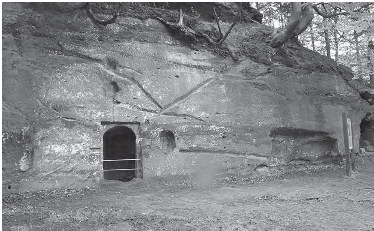
Fig. 15 - Wasigenstein: dripstone collecting the water along the cliff towards a cistern protected by a door. The water of the cistern was next drawn via this door and placed into a niche from where another dripstone led the water to the animal watering place.
