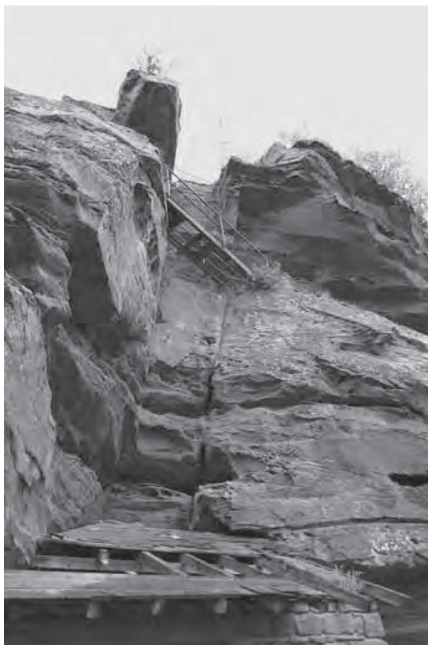
Fig. 20 - Falkenstein: rising column of the hoist crossed by the stair.
