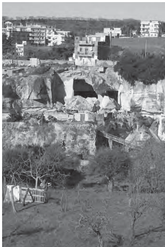
Fig. 9 - The fallen access to the underground quarry at Ginosa in Puglia (event no. 36 in Table 1). Note the proximity of the three-stories building to the sinkhole.
