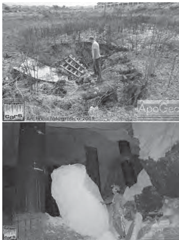
Fig. 3 - A sinkhole at Altamura, and an example of the failures in the underground system of quarries (photos by Centro Altamurano Ricerche Speleologiche).
