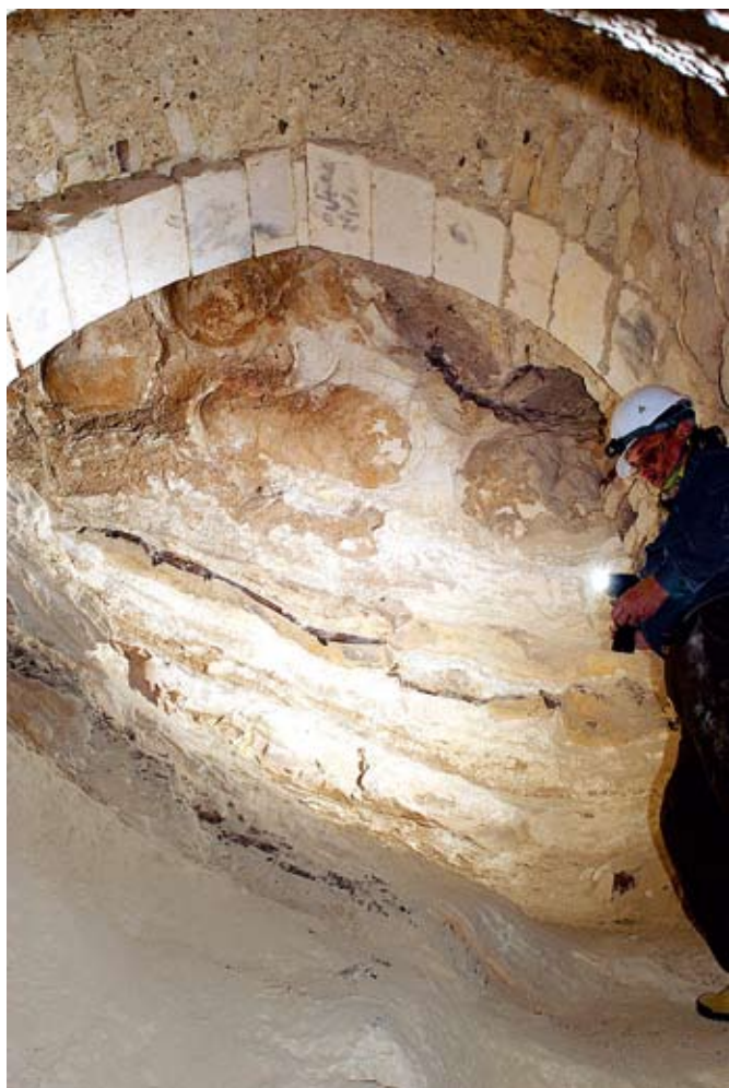
Fig. 9 - Part of the masonry supporting the helical section (photo C. Germani, E. Burri).
