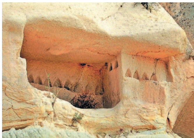
Fig. 6 – Kozanağa Mevkii (Göreme). Dovescote cut by the collapse of the external rocky wall that has put in sight the triangular niches for the nesting (photo A. Bixio).
