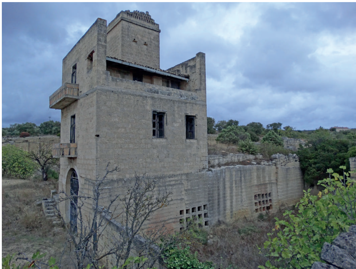
Fig. 2 – Casino Plasmati: an example of a Modern-Era semi rupestrian structure on a flat terrain. The walls of the ground floor are entirely shaped out of the rock (beehives grids are visible on the wall) and an entirely built floor is grounded on top. Antros Archive.
