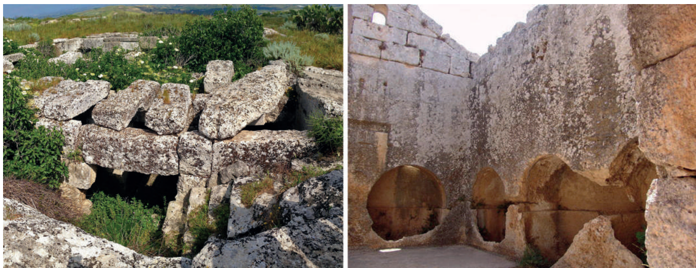
Fig. 6 – Example of the technique in other areas of the world: Colonne di San Basilio in Lentini on the left and Saint Simeon in Syria on the right. Ph. Franco Dell'Aquila.
