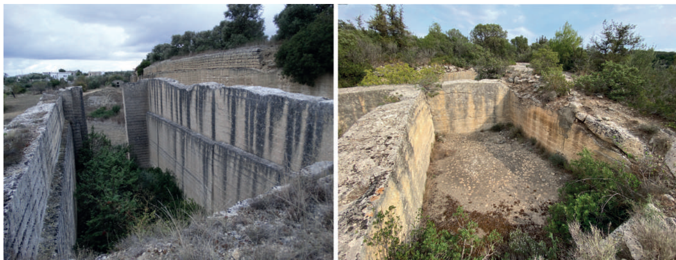
Fig. 1 – Uncompleted structures of the Modern-era semirupestrian technique of Matera: on the left an example on a flat terrain (at Casino Plasmati) and on the right an example on a slope (not far from Casino Passarelli) Antros Archive.
