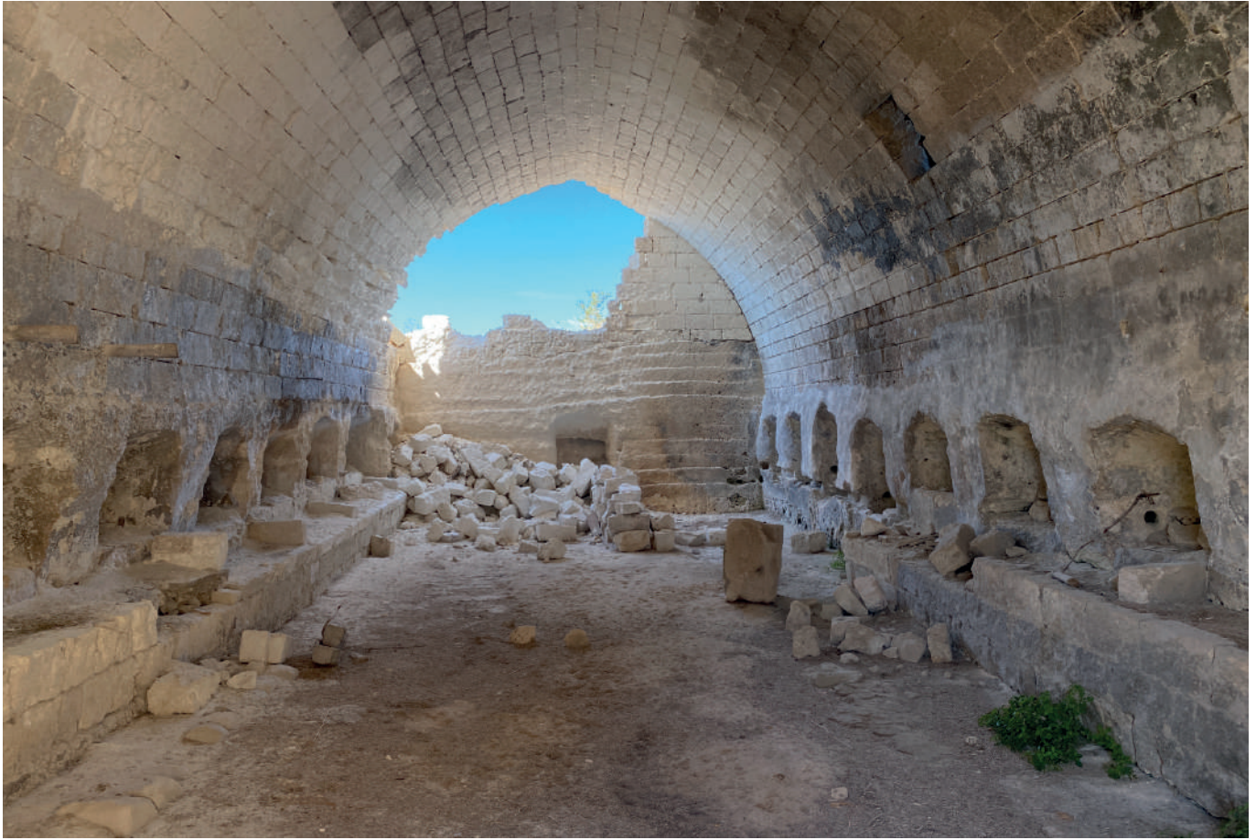
Fig. 4 – Masseria del Cristo, an example of the Modern-Era semi rupestrian structure on a slope, with the side wall entirely shaped into the rock. The built part of the back wall partially collapsed, highlighting the mixed type of architecture. On the side walls the mangers have been dug into the rock. Antros Archive.
