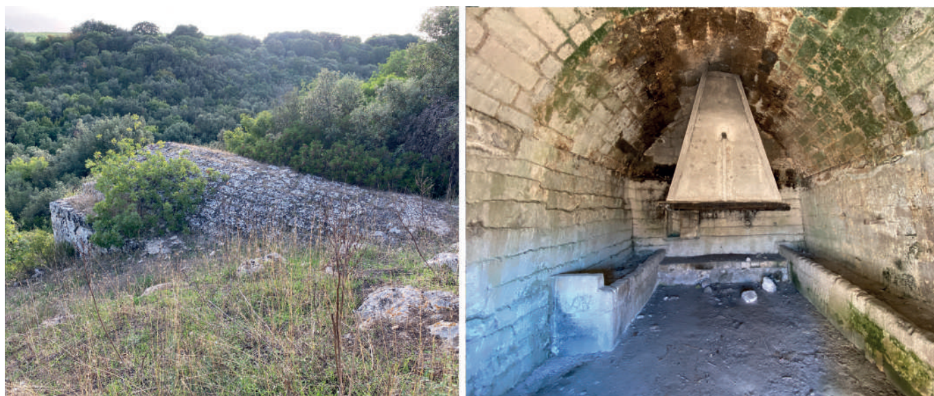
Fig. 3 – An example of the Modern-Era semi rupestrian structure on a slope, with the back wall entirely shaped into the rock. On the left lazzo di San Bruno, outside. On the right, Masseria Selva Teresa, inside. Antros Archive.
