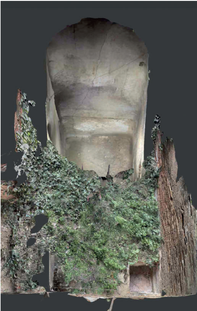
Fig. 6 – Irregular vegetation and square vertical cistern access (from above).
