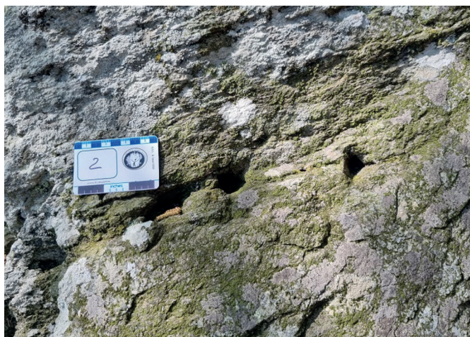
Fig. 2 – Denting left by pre-industrial rock splitting techniques (photo GGBV and GSL).
