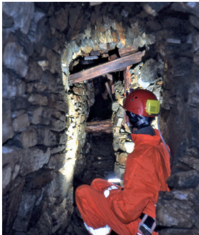
Fig. 4 – Kreas mine, Santo Spirito adit: the rock compression that has narrowed the tunnel (photo Paolo Testa).
