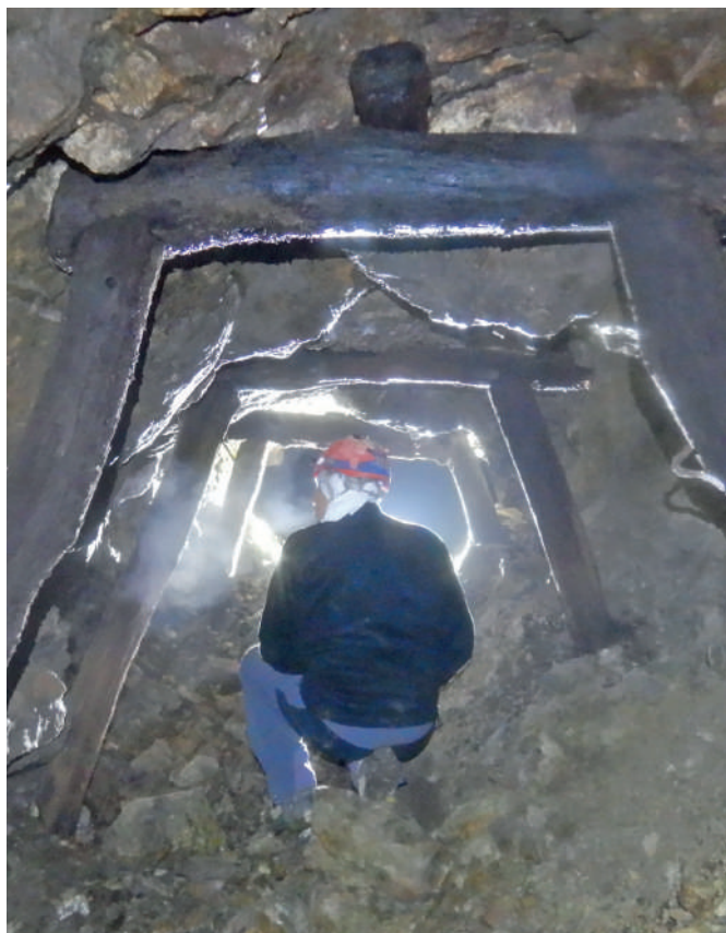
Fig. 8 – Costa del Ferro mine: recent timber support structures in an ancient, enlarged gallery (photo Paolo Testa).
