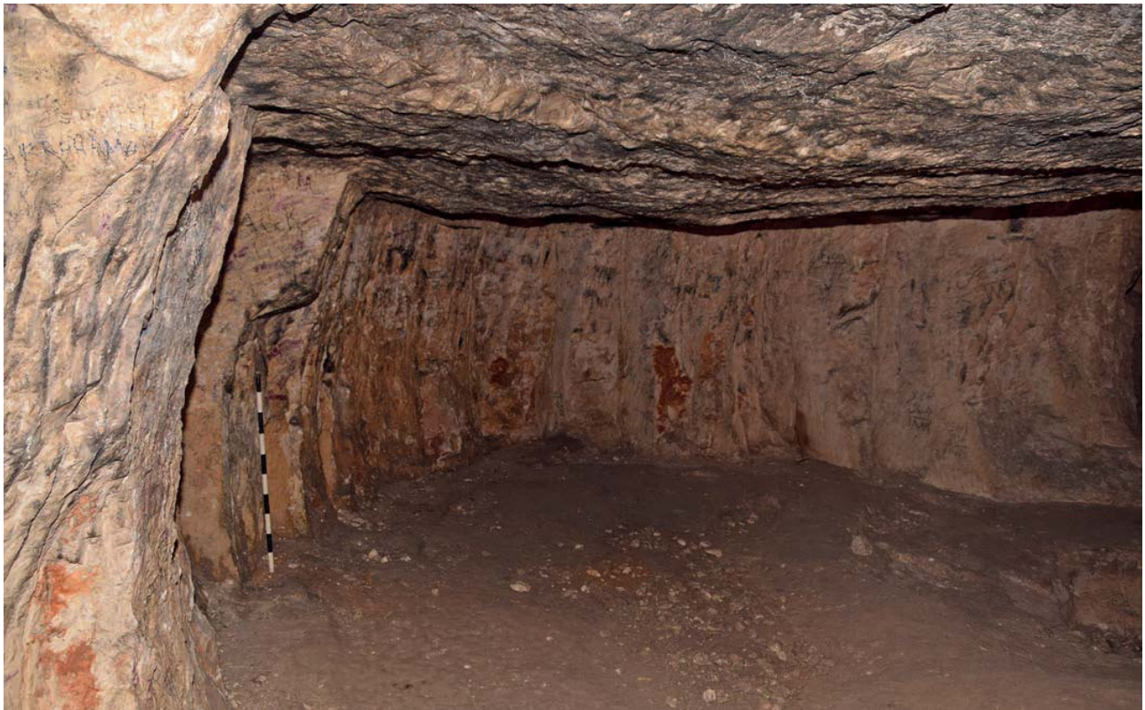
Fig. 6 – Remains of the column method of quarrying (photograph: Avraham Sasson; photograph 20/304).
