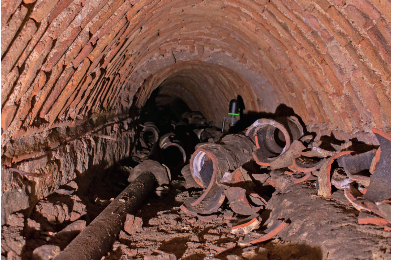
Fig. 2 – Leica BLK360 Camera Laser Scanner scanning in the tunnel (photo Özlem Kaya).
