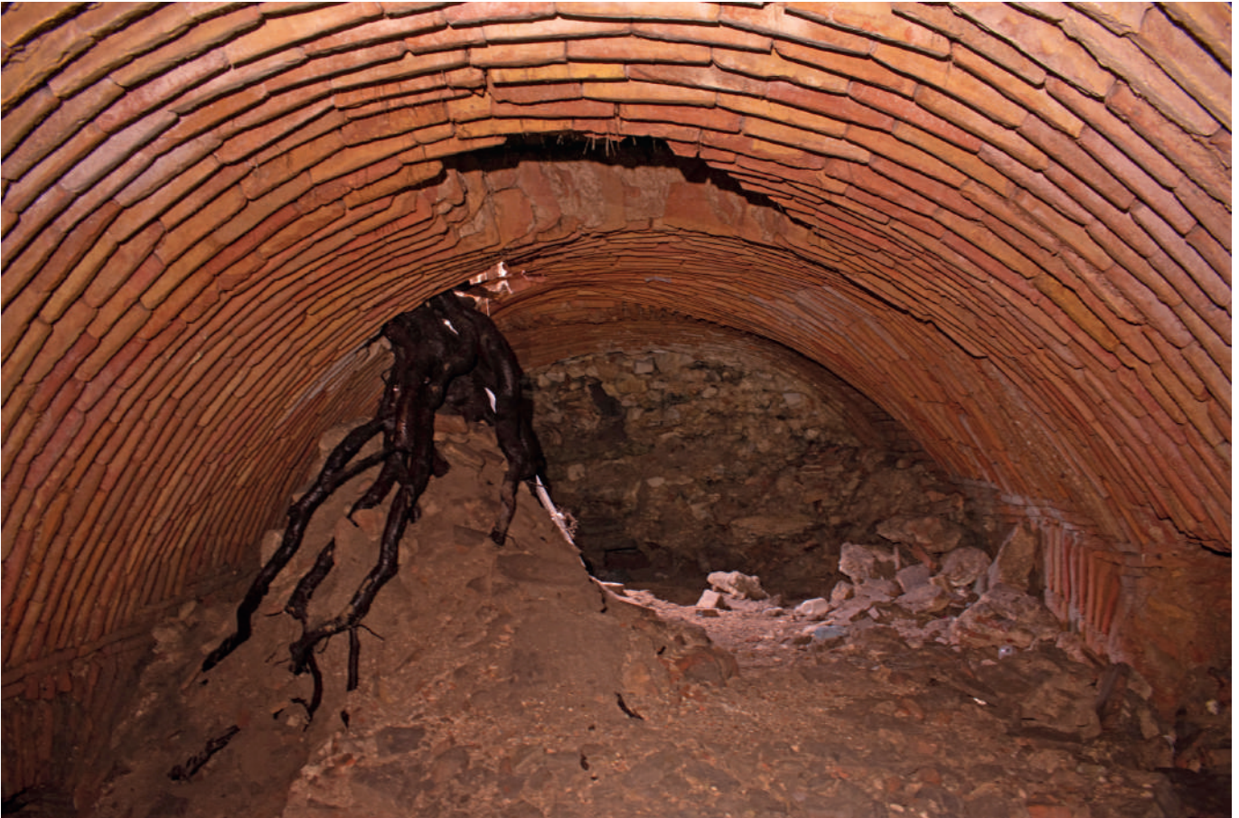
Fig. 6 – Brick arrangement in the tunnel (photo Özlem Kaya).
