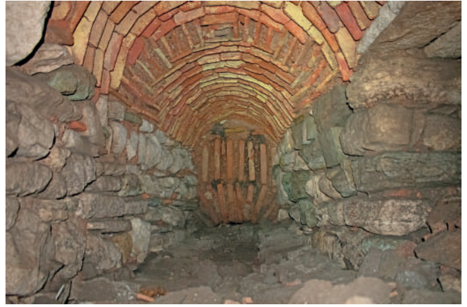
Fig. 5 – Roots of chestnut tree and the underground structure (photo Özlem Kaya).
