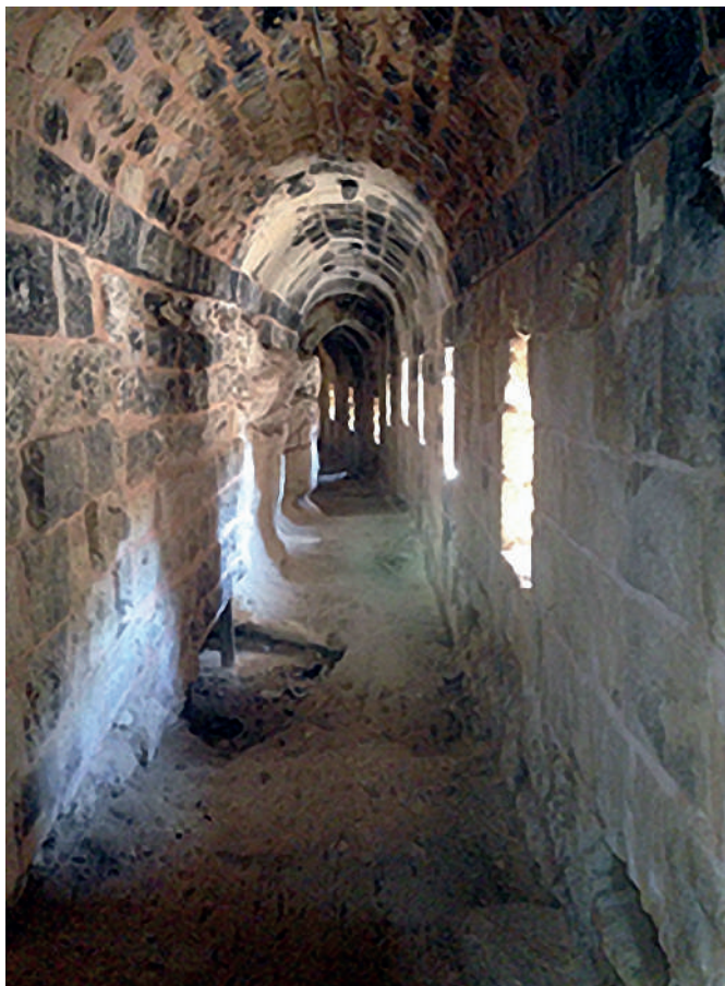
Fig. 6 – Defence gallery at the southwest side of the hill (photo A. E. Keskin).
