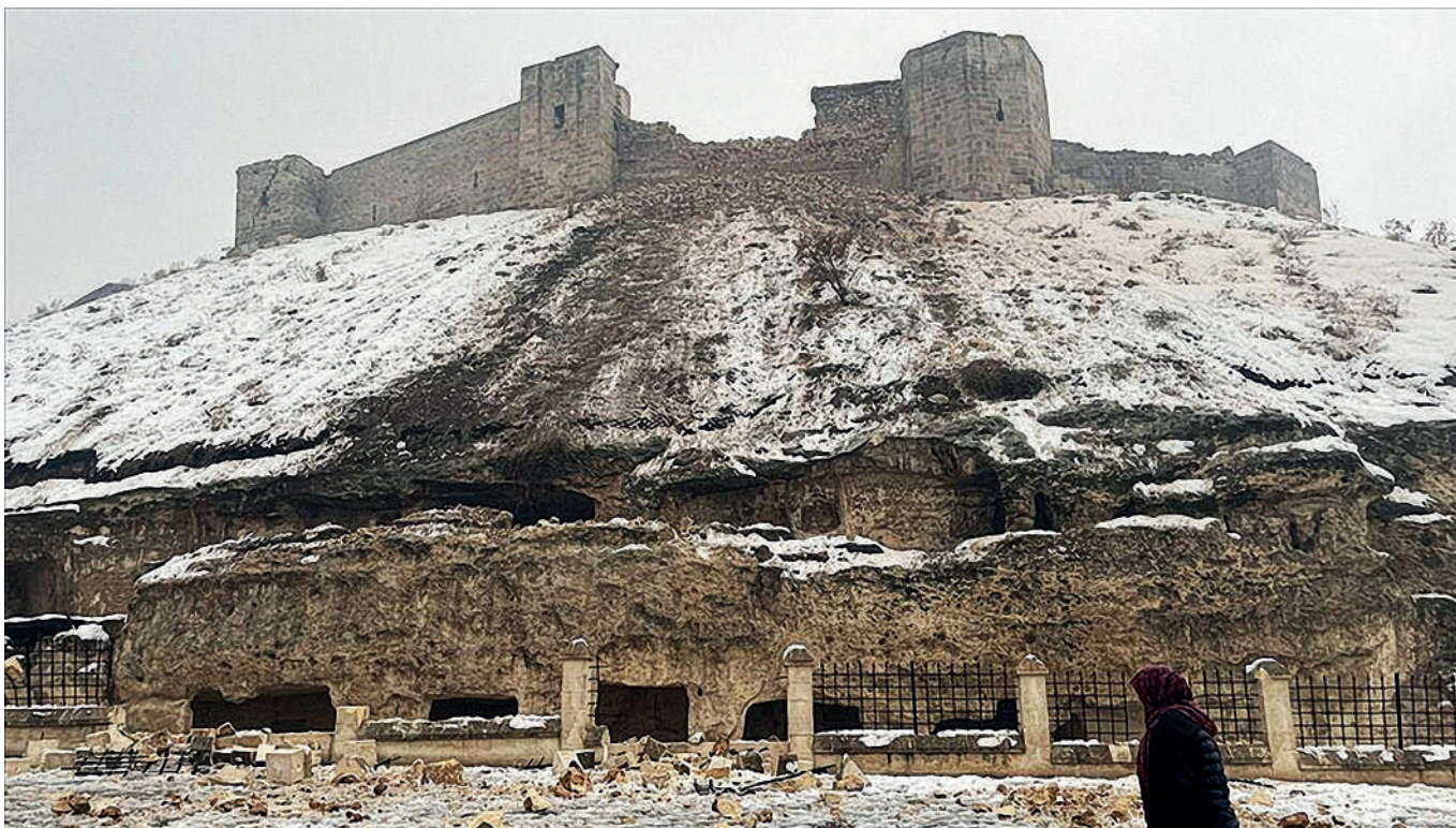
Fig. 7 – Destruction and erosion at the east side of the castle after the February 6, 2023 earthquakes. Some of the dwellings can be seen at the foot of the hill (photo E. Ozihtiyar).
