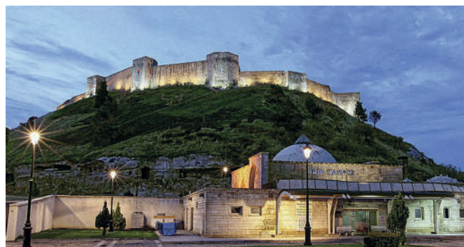
Fig. 2 – Gaziantep Castle before the February 6, 2023 earthquakes. View from the northeast (photo S. Savcılı).
