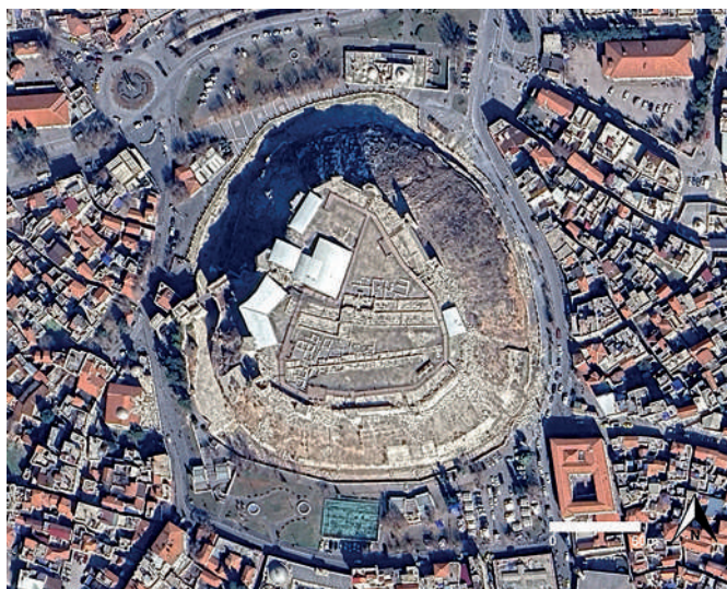
Fig. 3 – Aerial view of Gaziantep Castle (Google Earth).
