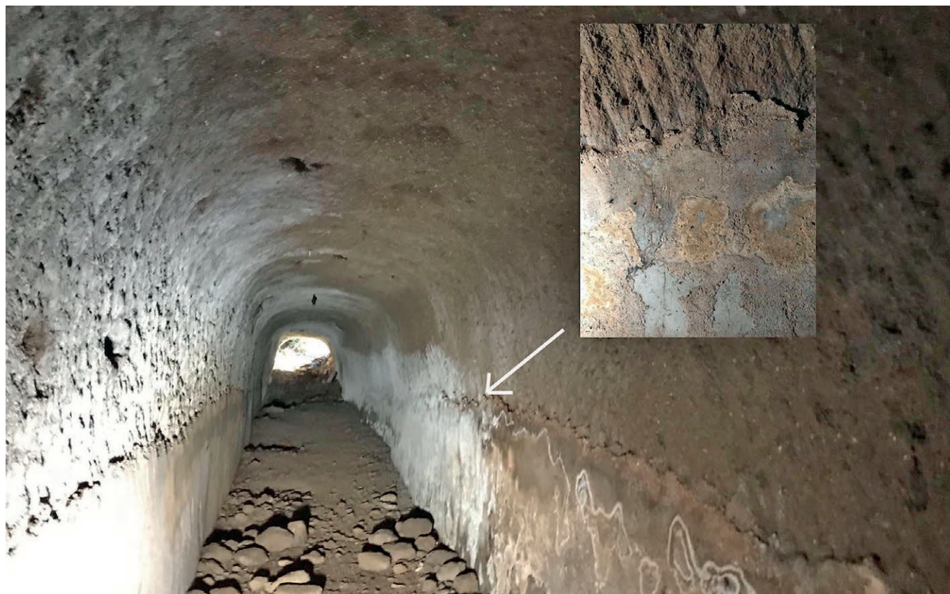
Fig. 6 – The detached branch E'', and detail of its plastered wall, with lime deposit above it and digging traces below the plaster (photo A. Schatzmann).
