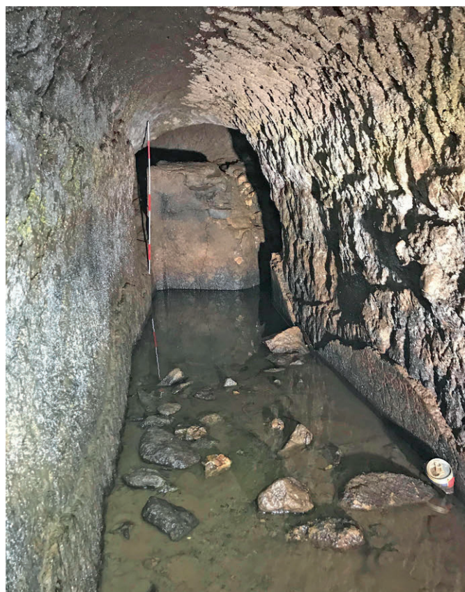
Fig. 7 – Intersection between conduit I and corridor G (from where the photograph is taken). The vertical quarter round is well visible in the left angle of wall H (photo A. Schatzmann).
