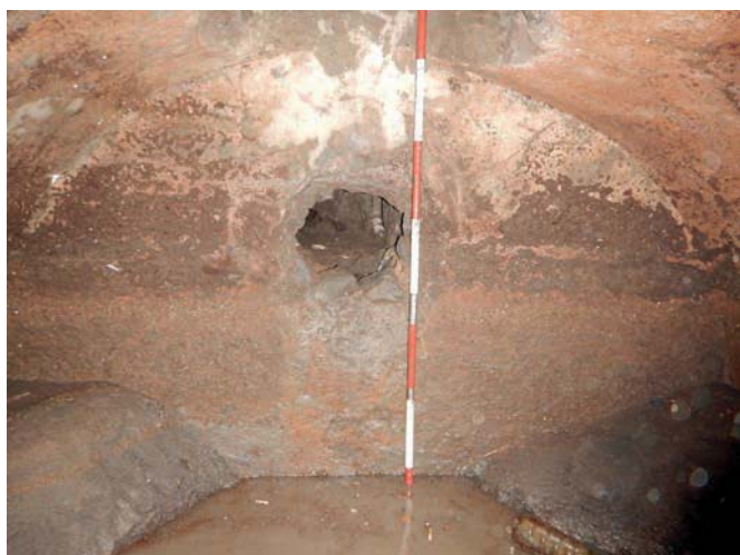
Fig. 3 – Pompeii, Civil Forum, south cistern: the western side and the intake hole (photo G. Ferrari).
