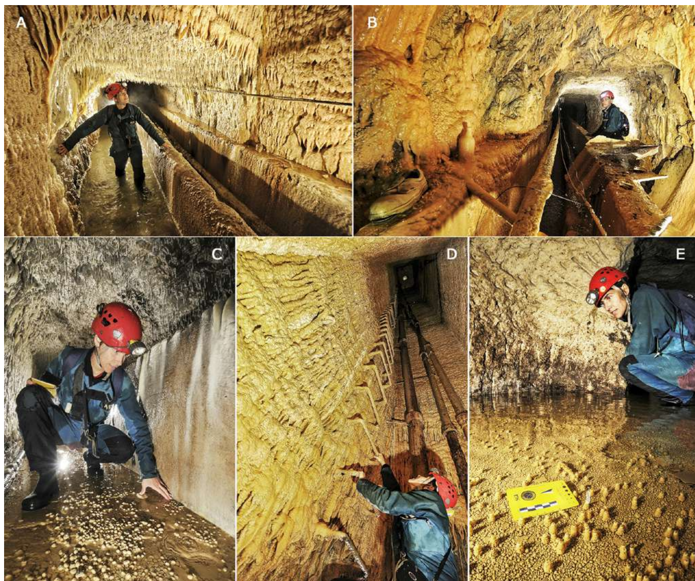
Fig. 2: main features of the Bunnari aqueduct. A: the adductor canal on the right side of the tunnel where water reaches a deep of 50 cm. B: the calcite coating covers walls, ceiling and any artefacts where the tunnel pass through calcarenites. C: white pisolites occur on the floor below few cm of water. D: the rectangular ascending chimney equipped with iron rungs. E: the niche where the anti-stalactites form (photo A. Romeo).
