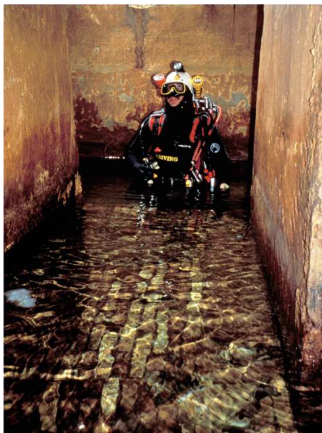
Fig. 12: the underground stream interception of the Domusnovas aqueduct (Sardinia) connected to the "Su Stampu de Pireddu" cave spring (photo Marco Vitelli).
