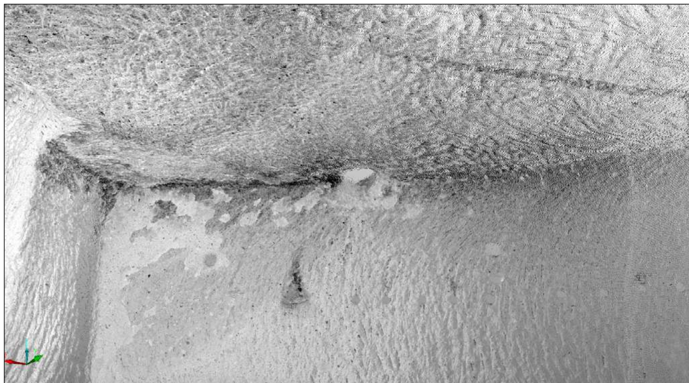
Fig. 2: Göreme, Aynalı Monastery, NE room, detail of the cloud of points. In the middle the hole of an aeration conduct connecting the room with another room two levels above. On the walls the pseudo-circular carved traces of excavation are shown (image by M. Carpiceci).
