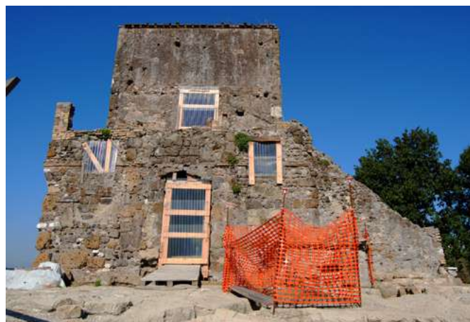
Fig. 2: the tower view from the east with the entrance and the staircase added in the second phase.
