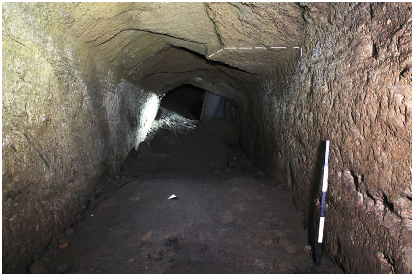
Fig. 12: tunnel track between B and C. The original ceiling is indicated (photo V. Puggini).
