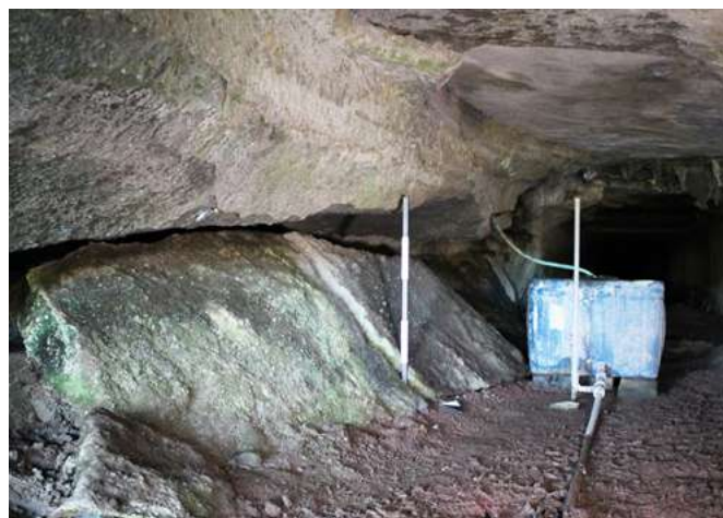
Fig. 10: detail of the collapsed N wall between cuniculus and tunnel (photo V. Puggini):
