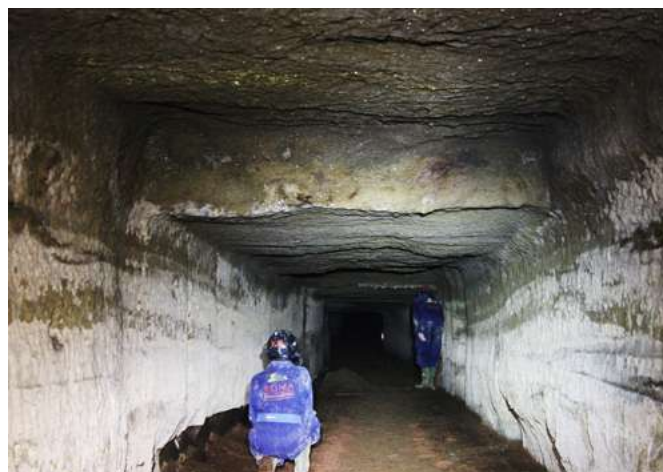
Fig. 8: not standardized step in the ceiling (photo V. Puggini).
