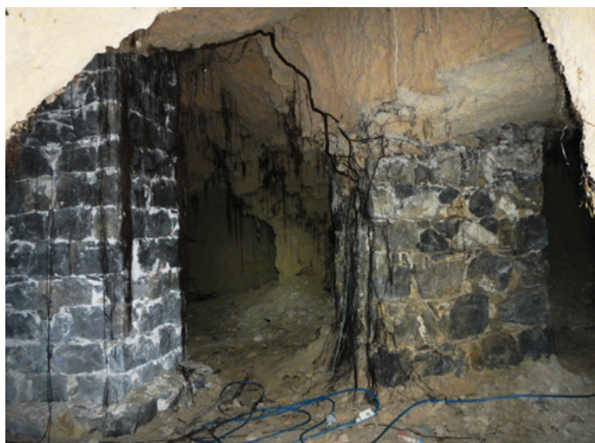
Fig. 9: the wide central volume of the underground quarry is sustained by two massive pillars made by cemented rocky blocks (see figg. 7 and 8 for location).
