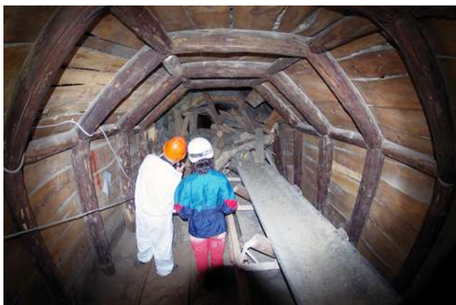
Fig. 2: the "Floatation" tunnel during inspections of May 2014 (photo G. Badino).
