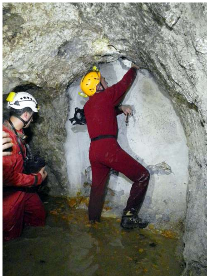
Fig. 10: the 3 th level gallery which ends on the gypsum blocks man-made wall. Over this the passage is blocked by the debris deposit (photo M. Vattano).
