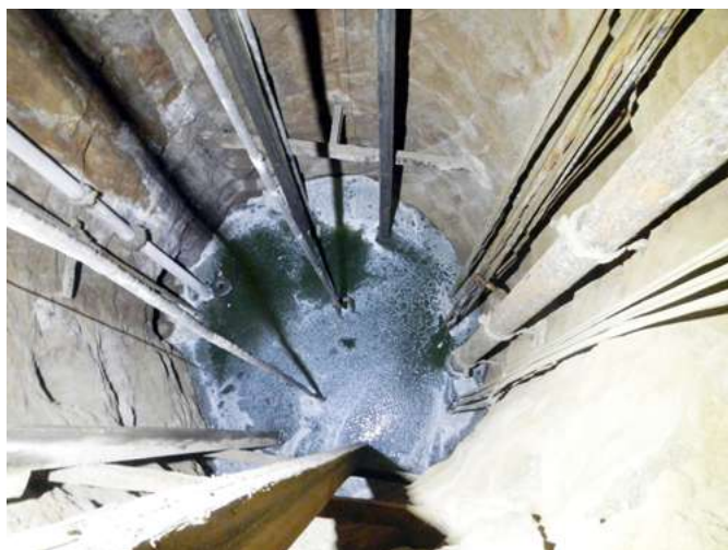
Fig. 4: view of the Main shaft, from the 5th level gallery, in 2014 May (photo M. Vattano).
