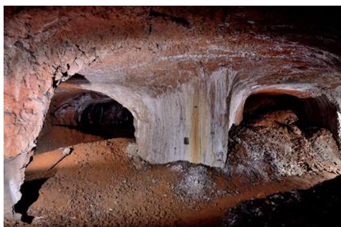
Fig. 6: support pier carved by excavators (photo M. Gradozzi).
