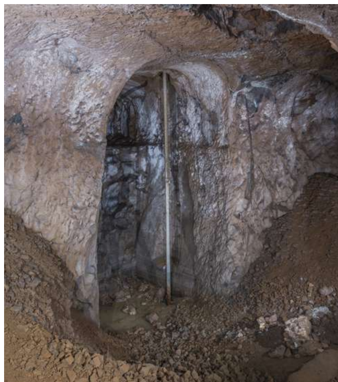
Fig. 10: modern well pipe tapping the aquifer (photo M. Gradozzi).
