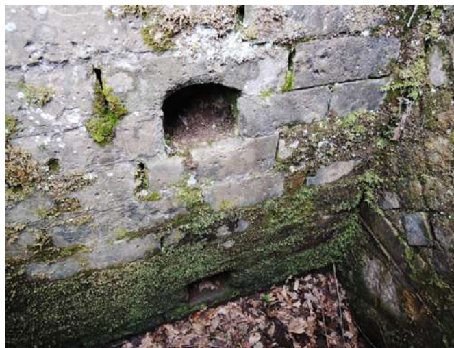
Fig. 13: the footholds made by special bricks (photo V. Colombo).
