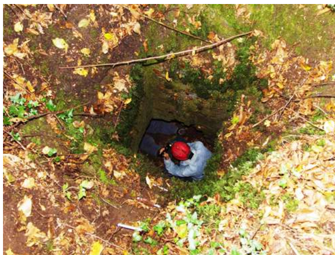
Fig. 12: a deep wells: the tunnel is accessible from the base of the shaft, passing the pile of debris (photo C. Germani).
