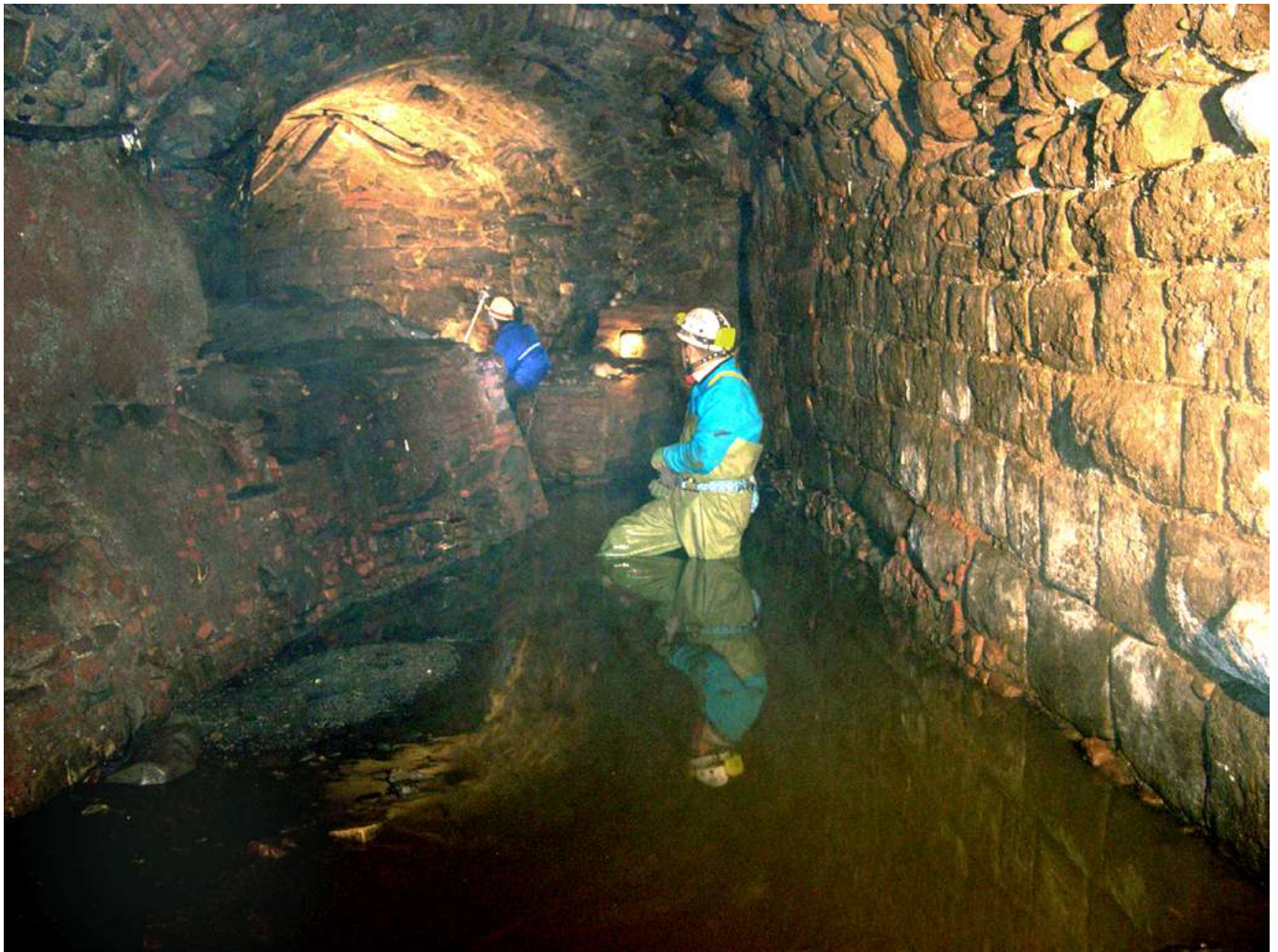
Fig. 9: wall with bossed stone masonry (photo R. Bixio).
