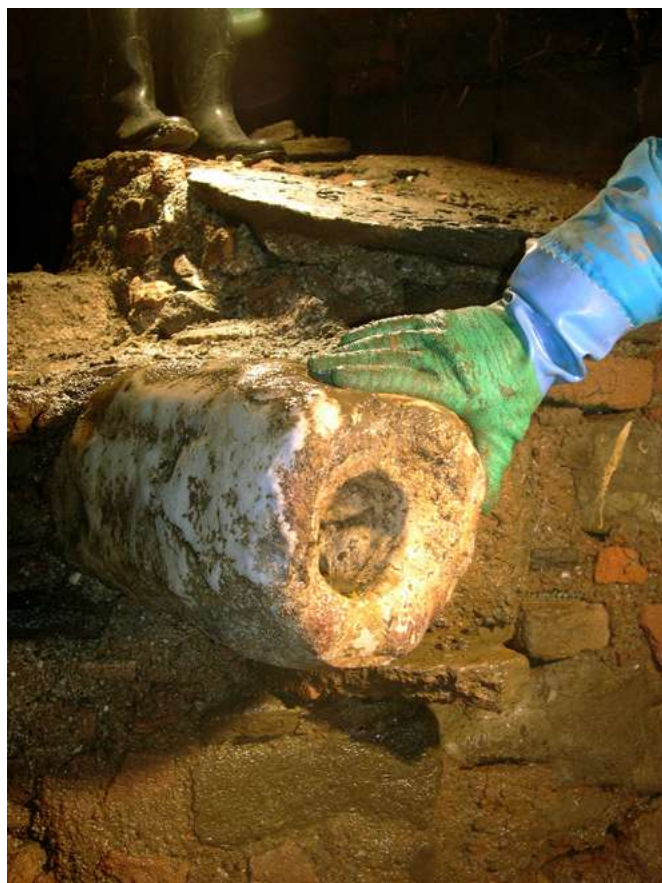
Fig. 13: detail of the marble pipeline of the ancient aqueduct still incorporated in the main wall (photo R. Bixio).
