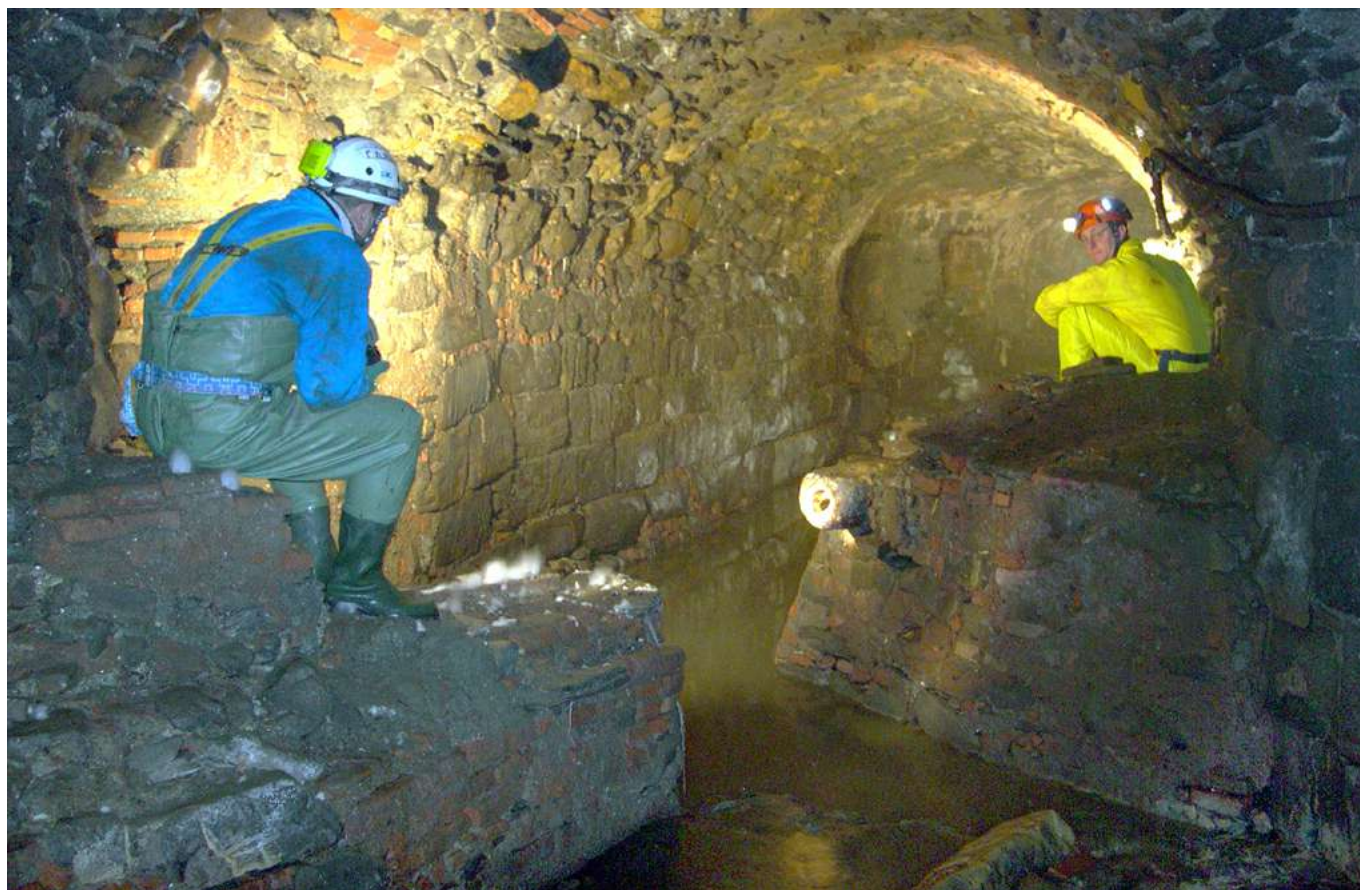
Fig.12: pillars holding up the marble pipeline of the ancient aqueduct that crosses the streambed (photo R. Bixio).
