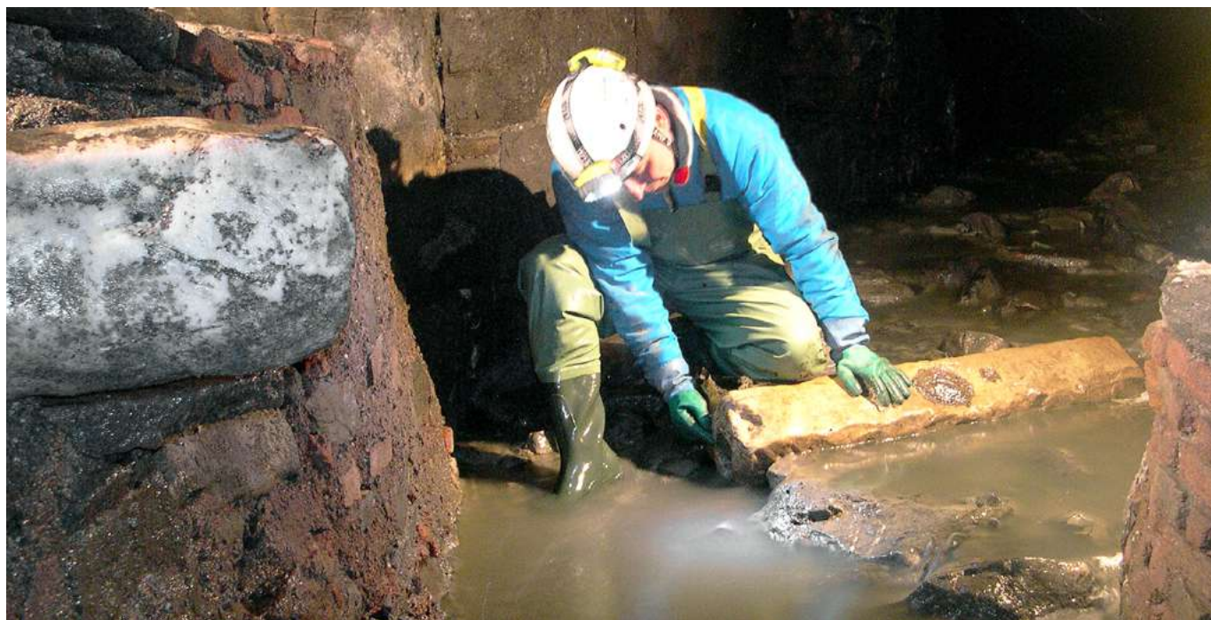
Fig. 14: aqueduct's marble element removed by floods from its suspended original position (photo R. Bixio).
