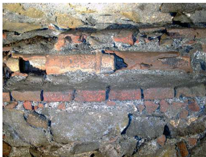
Fig. 11: ancient clay tubes incorporated in the lateral wall of the tunnel (photo R. Bixio).
