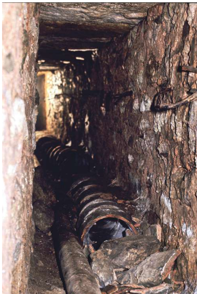
Fig. 2: the gallery with terracotta and iron pipelines (photo Metin Albükrek).
