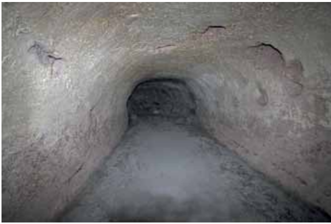
Fig. 5 – A large basket vaulted gallery in the southeast section of Derevank Monastery (photo A. Yamaç).
