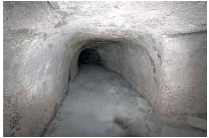
Fig. 9 – The large straight basket vaulted gallery, 21 m long, which connects to the church (photo A. Yamaç).
