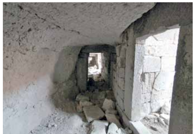
Fig. 10 – The doors of the chambers along the longitudinal flat-ceilinged corridor (D). One can note the walls partially composed of squared stones, as well as jambs and lintels made from monolithic blocks (photo A. Yamaç).
